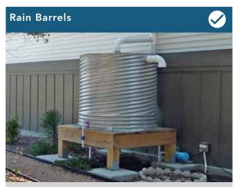
Rain barrels are storage devices that collect rain water for reuse in lawn and garden watering or other uses. They are generally connected to roof gutter systems.
