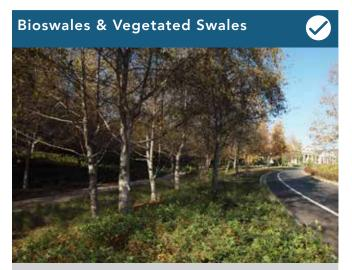
Bioswales and vegetated swales are linear bioretention systems used to partially treat water while also conveying flows to larger bioretention or other stormwater management systems.
